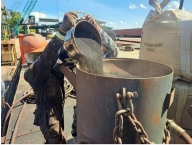
Figure 4. Put copper slag into the sandpot
